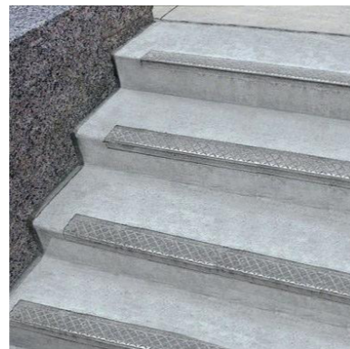
Insitu concrete steps
