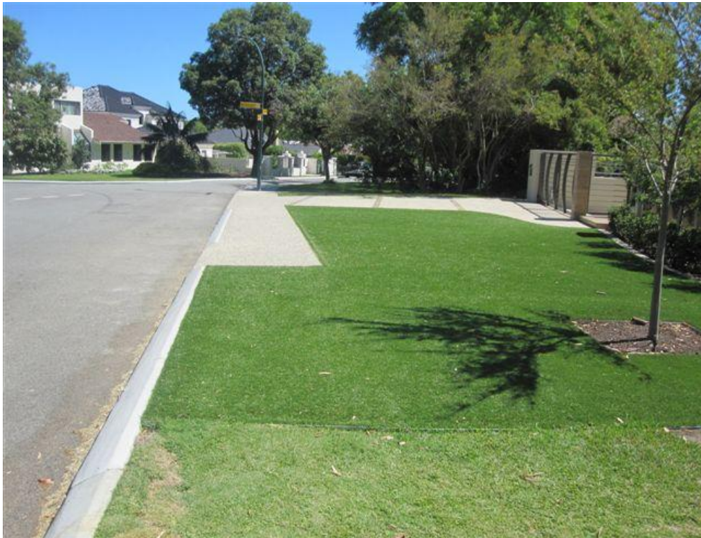
Figure 1 – Verge area showing extent of artificial grass
