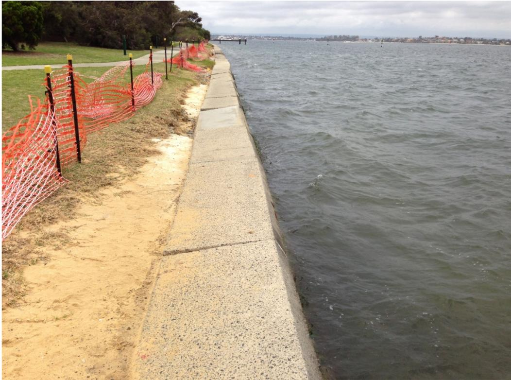
Figure 3. Damaged Wall and Temporary Fencing
