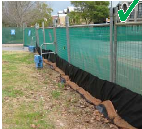
Secure the geotextile material to the perimeter fence to a minimum height of 600 mm.
